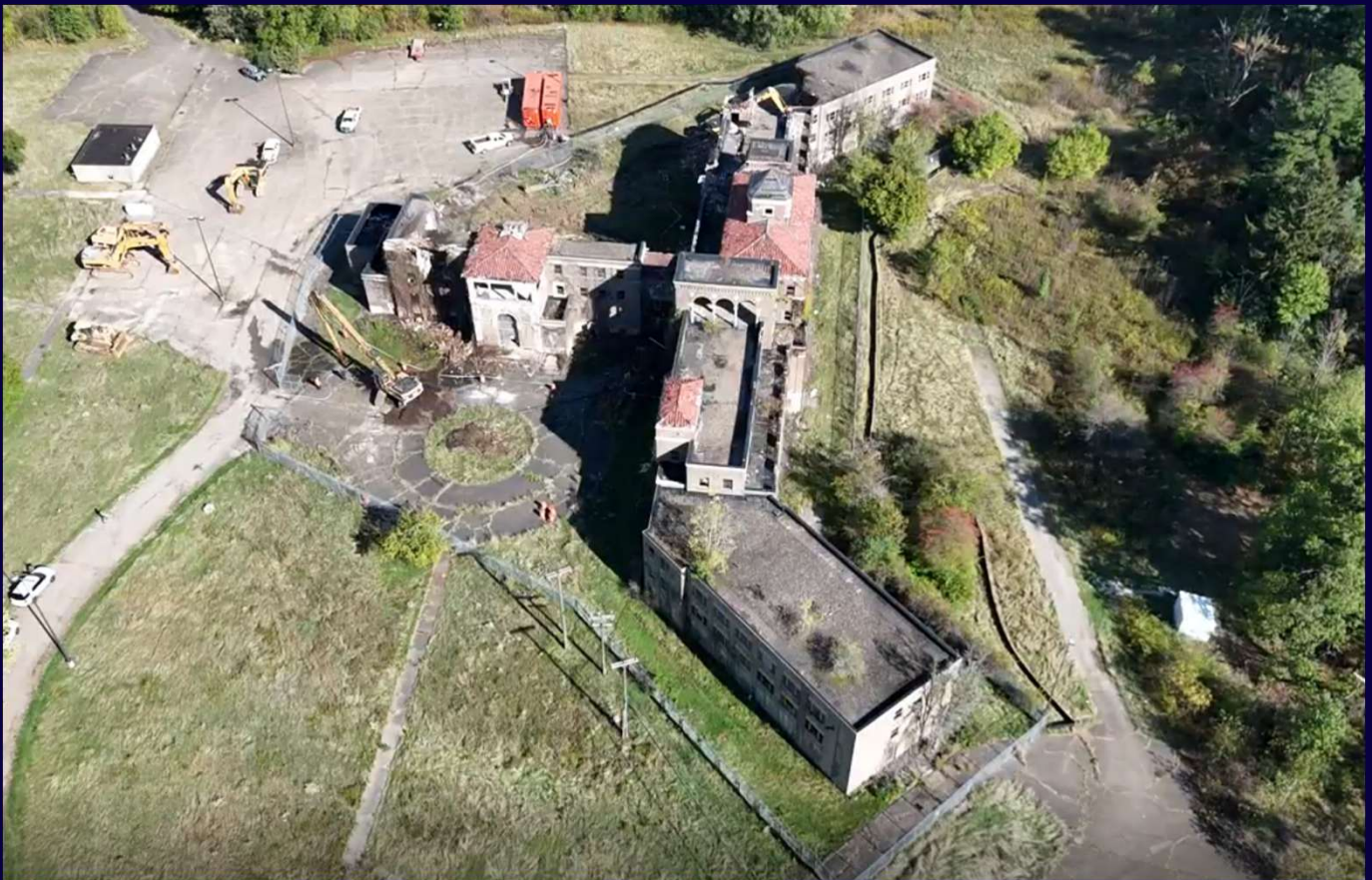
Drone image during early demolition of the main building
